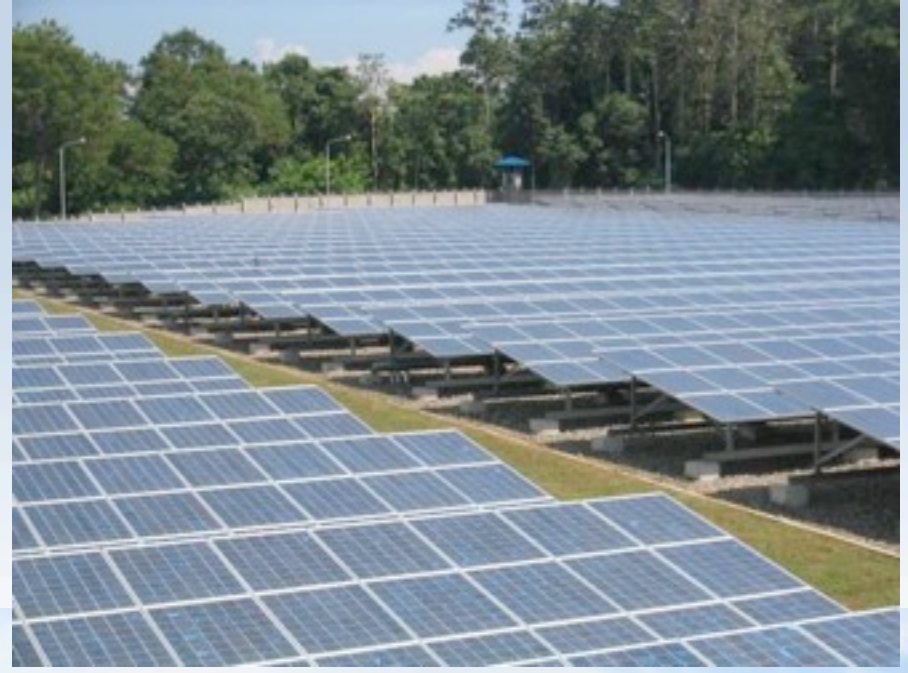
Expect fixed mount multicrystalline solar panels and small scale demonstration of next generation technologies
